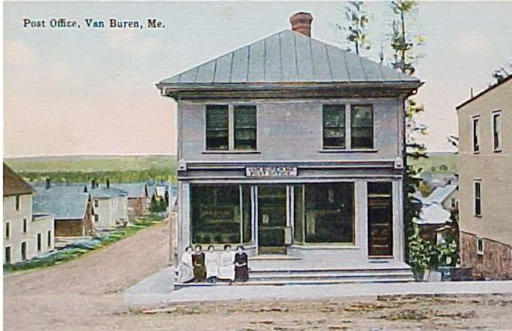
Post Offices at Van Buren (above) and South Gardiner (below).
